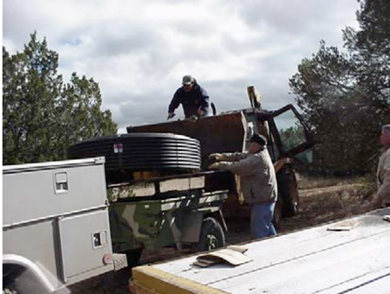
Fort Stanton Water Main Installation – 2002
