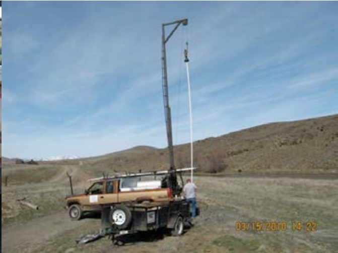
Installing the pump at the new Presley Trailhead. Note hitch rails and permanent toilet in background.
