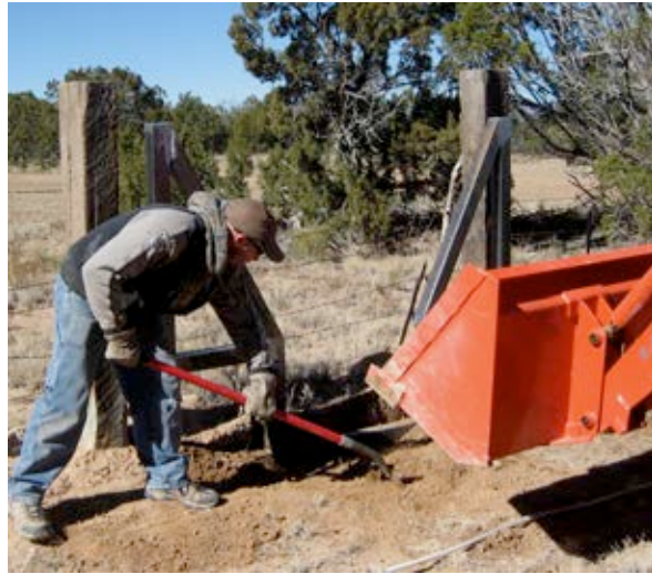
Trailhead Gate Installation
