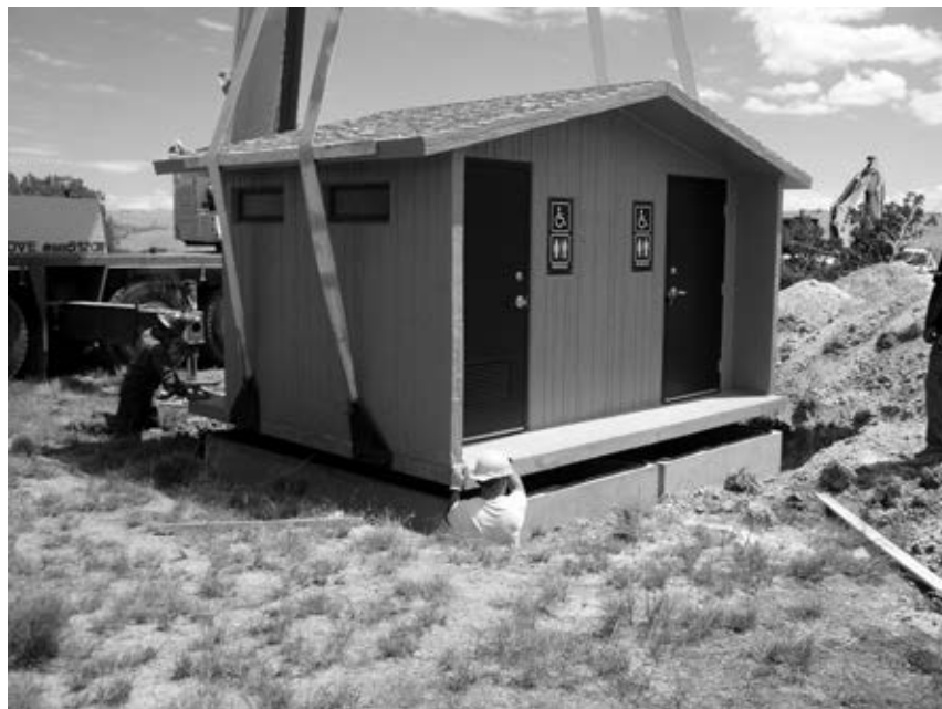
New Toilet Installation
